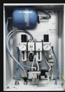
Air Treatment Unit (valves, filters, buffer vessel)
